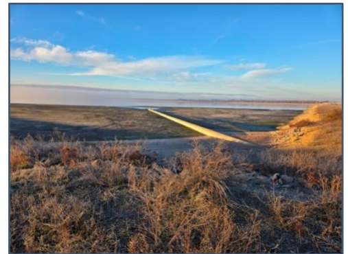
Low water at the Muskegon wastewater facility (Don Burlett)
